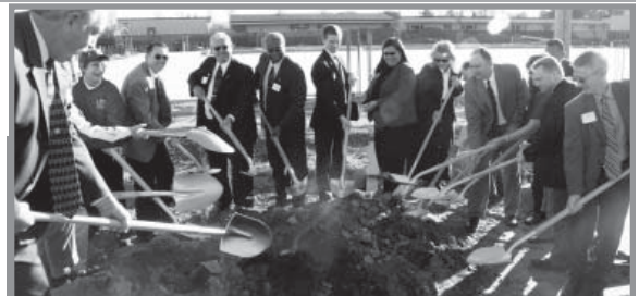
Lodi Unified School District representatives break ground for Lodi High School's new cafeteria and gym
